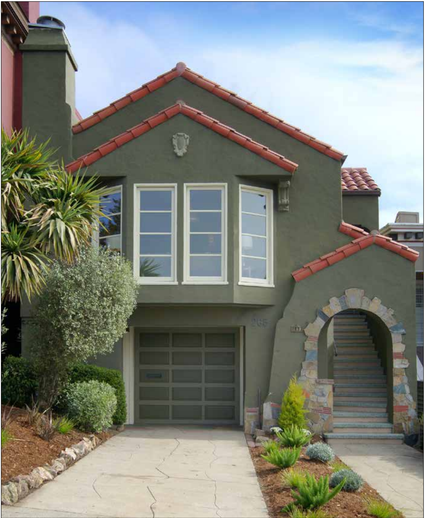
265 CLAREMONT BOULEVARD, SAN FRANCISCO SOPHISTICATED REMODEL ONE BLOCK TO WEST PORTAL VILLAGE
